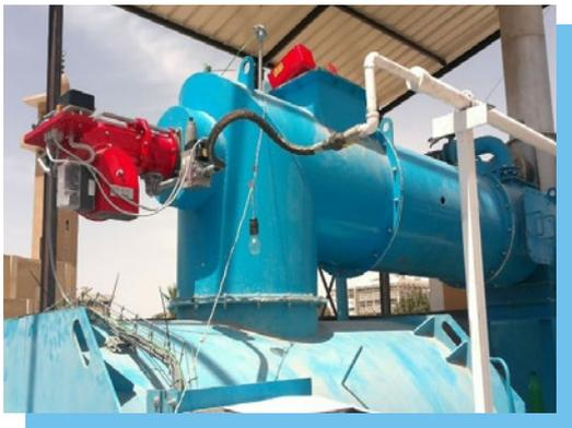
Post-combustion filtration results from the oxidation of gases from the combustion chamber. The dust contained in the fumes is partially eliminated at the same time as the microparticles contained in the fumes. Post-combustion, placed under the combustion chamber, completes the oxidation of fats, a process initiated in the combustion chamber.
